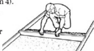
(Diagram 4 - Screeding the sand)
